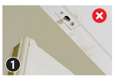
Check that the door fits the frame properly. Excess friction or scraping between the door and frame can cut the line. **DO NOT USE** if corner of door scrapes against the frame.
